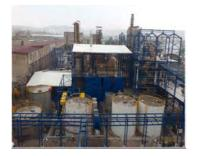
Description: Providing Engineering, Procurement and Construction services to Design and Build a Potassium Nitrate Fertilizer (NOP) Plant with a production capacity of 50,000 metric tons per annum in the IGSAS Fertilizer Complex.
